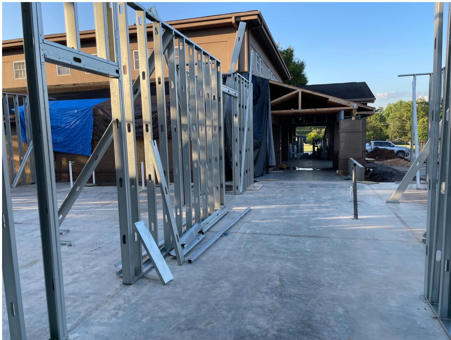
IMAGE #6 - Down New Hallway with Admin Offices to Left
